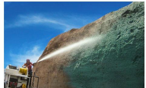
Figure 1 HECP being sprayed onto a steep slope
