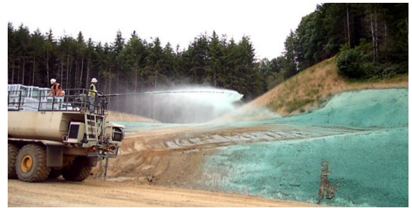
Figure 2 HECP being sprayed onto a sloped surface
